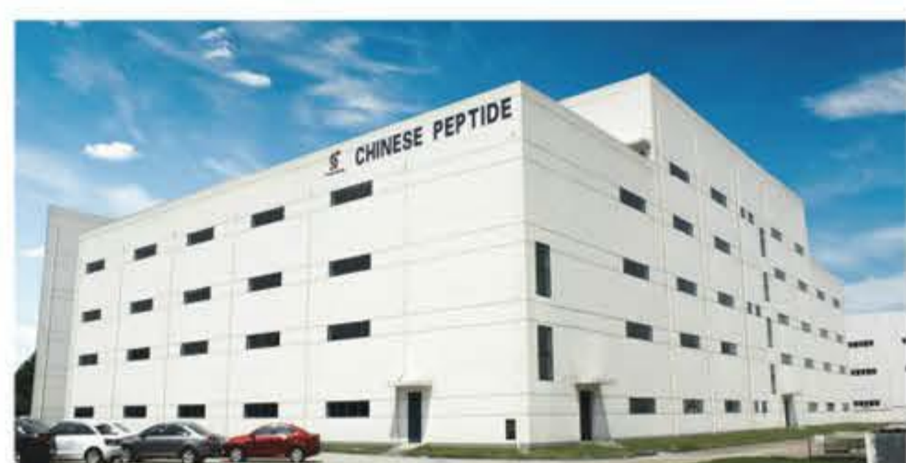
Headquarter & Manufacturing Site
